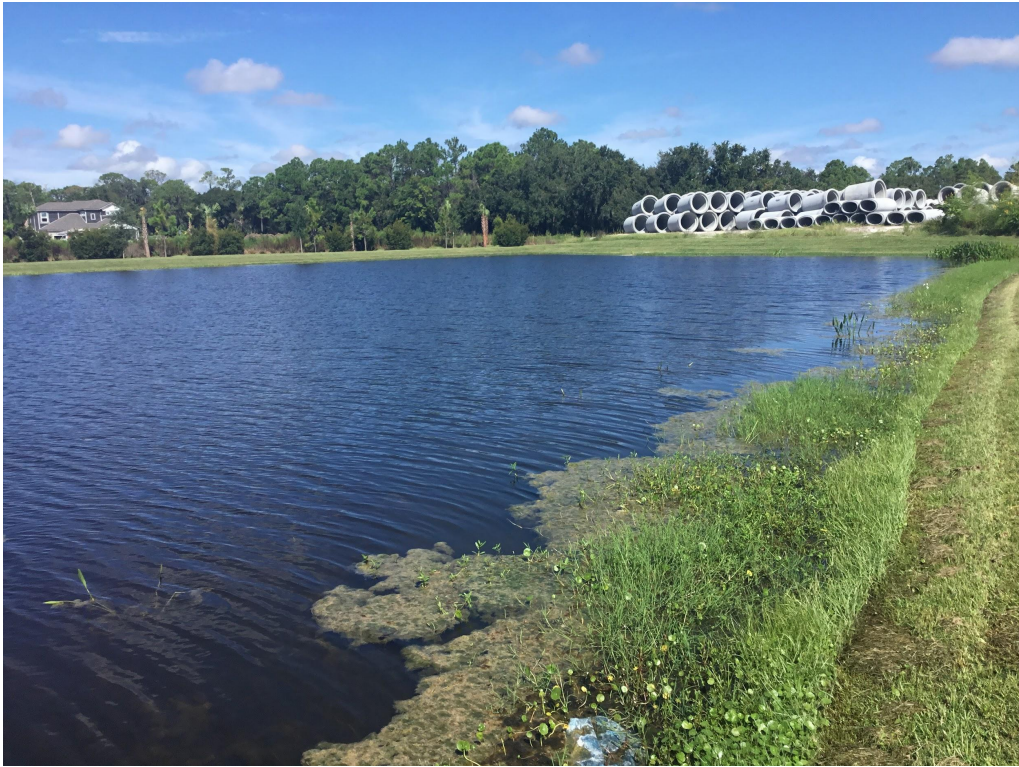
Photo 17: Taken from Photo Station M, site 3, facing northwest.
